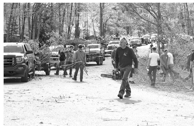
Volunteers create plans and work together to clean up Shady Brook community downed trees after Friday's deadly tornado. Photo by Joanie Moore.
