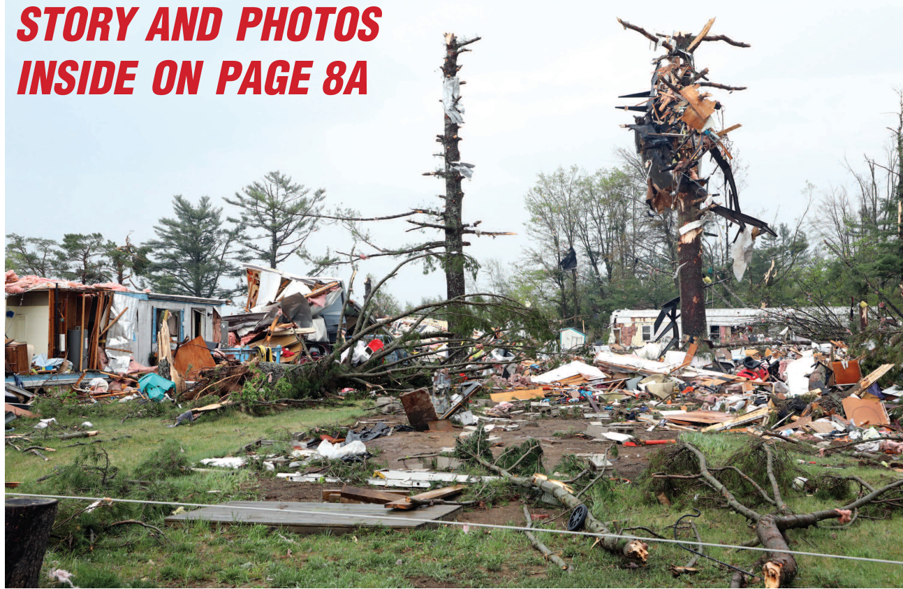
Mobile homes in the Nottingham Forest manufactured home residential community were flipped over and torn open during Friday's tornado, leaving many of the residents homeless. Parts of homes were thrown into the air, crashing down into trees and scattering throughout the park. Emergency first responders tended to victims, some of whom were taken to area hospitals. Photo by Joanie Moore
